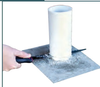
Cut the stub out as close to level with the floor as possible.
